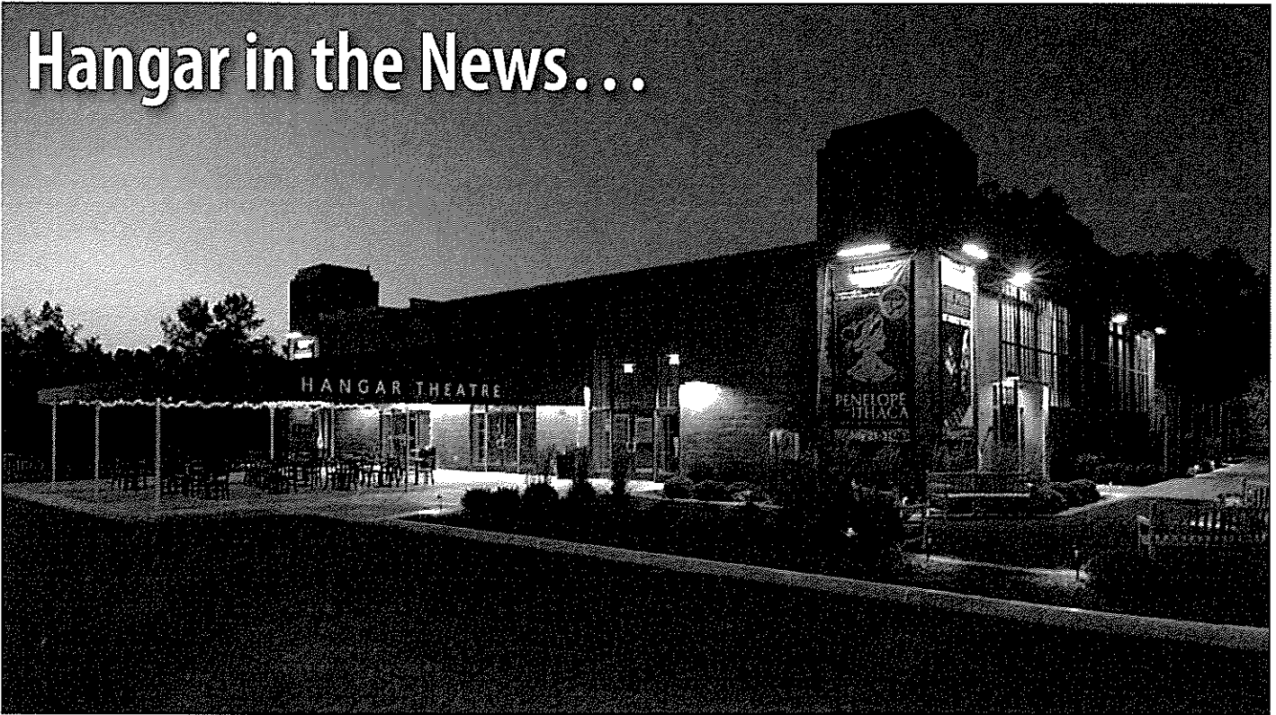
Our new home. Photo provided by HOLT architects.
